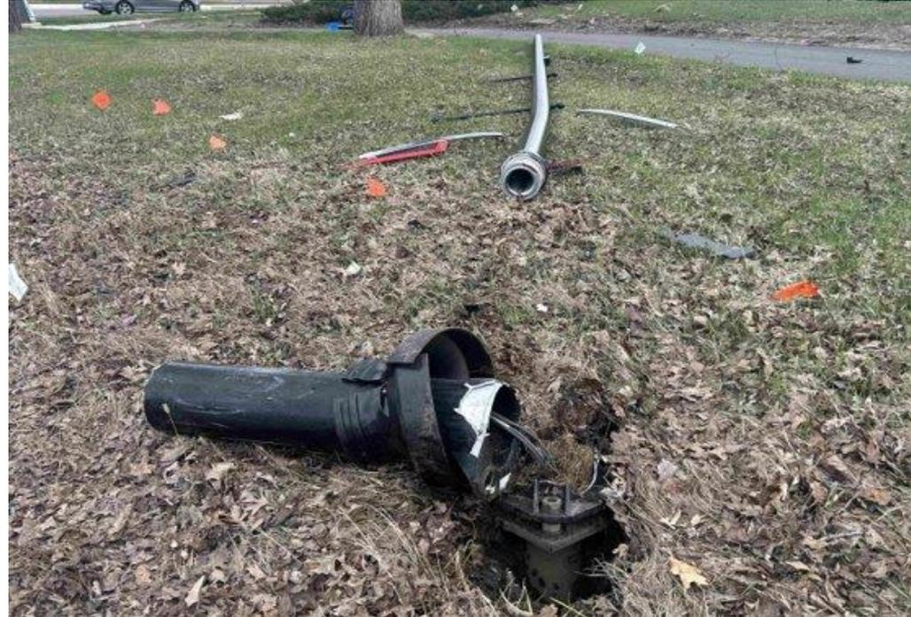
**When light poles are damaged, the underground wiring is not covered to/from poles.**
